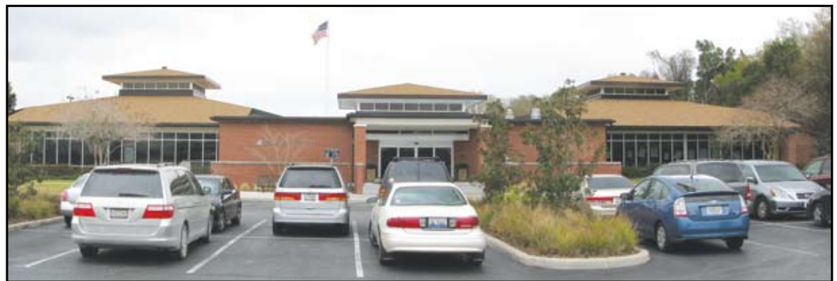
The wing added in 2007 on the right side of the Land O' Lakes branch is one of the few library construction projects in recent years in Pasco County.
